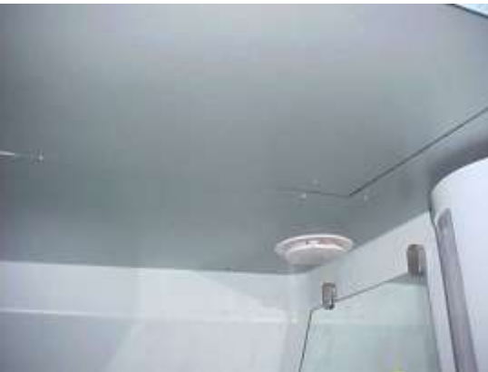
← “Alucobond” lavatory ceiling panel
